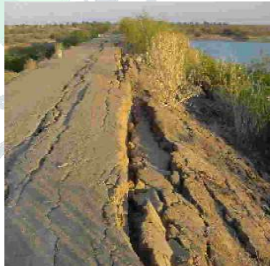
fig 2: failure of upstream crest of fategadh niigata, dam, (courtesy of iit kanpur)[1]
